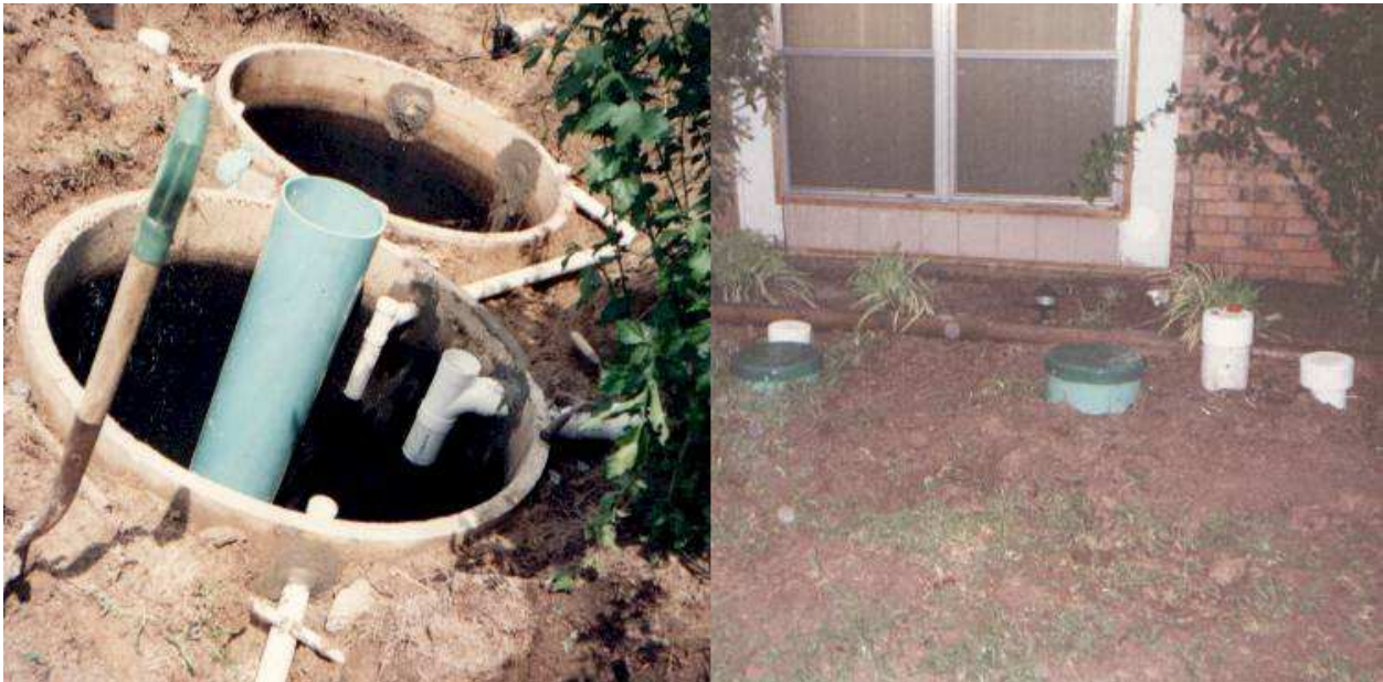
Figure 7. Conversion of a holding tank system at the Kolyts site.
