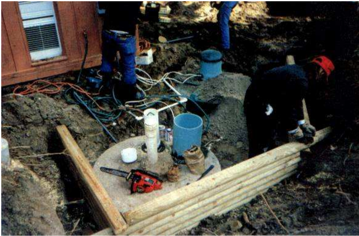
Figure 3. Innovative design for the Roy Walker site that corrected a 100% failed field and tank system using the existing tanks.
