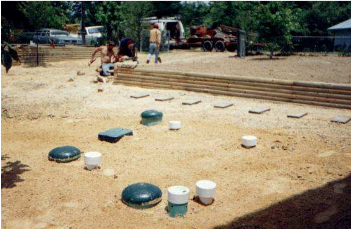
Figure 8. The Foster residence restoration of a holding tank system.
